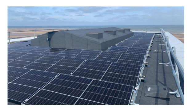
The project underway at **Betws Gwerfil Goch primary school** will show what can be achieved at sites not connected to the gas network. The oil boiler is being replaced with an Air Source Heat Pump. This is complemented by a solar PV array on roof and battery storage. The project will decrease the carbon emissions at the site by 7 tonnes per year.
