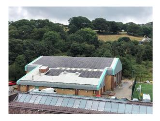
At **Pavilion Theatre**, **Rhyl**, there is now a 19.6 kW PV array on the roof. LED lighting is being installed in the auditorium and the project includes the upgrading of the boiler and heating and ventilation system. These will decrease the carbon emissions at the site by approximately 30% (173.2 tonnes per year).
